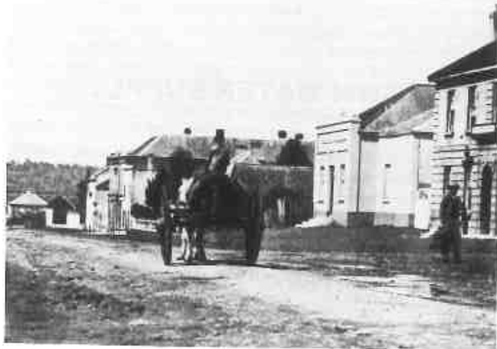
Town Water Supply.
